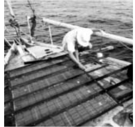
Work on the photovoltaic raft
